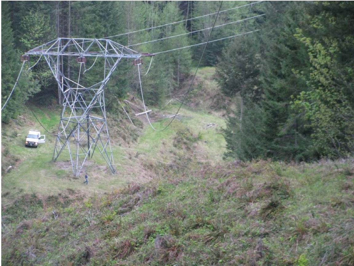
Figure 1 – Olympia _ Grand Coulee Str. 70/2 looking Back on Line
