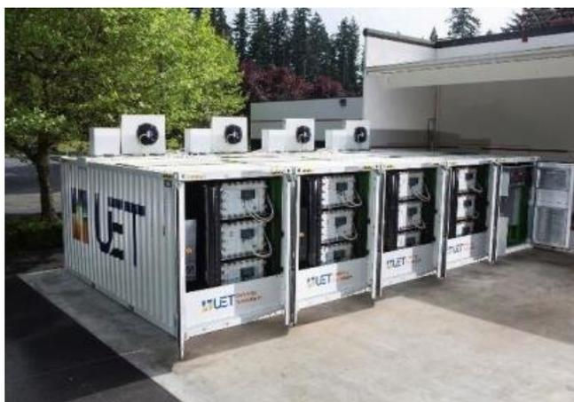
Not a substation, this battery at the end of two feeders, will also be used by Avista for grid control, load shifting, frequency and voltage regulation, Gibson said. A centralized controller that can optimize the assets.
